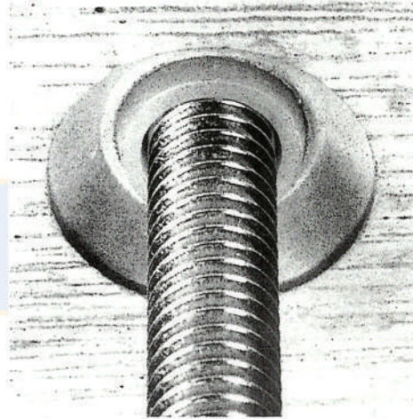
Good out-looking of concrete-surface
