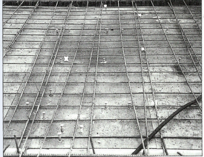
⑥ Disjoint the wooden formwork and set the bolt.
